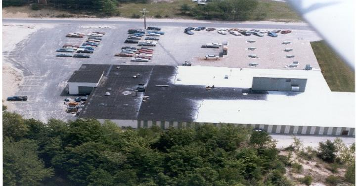
*The Bluestone Super Duty Aluminum paint reflects UV rays and lowers the temperature of the roof.*
