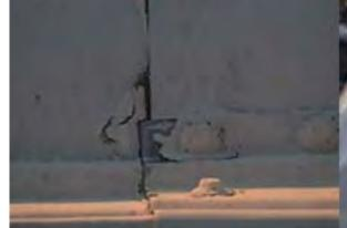
Previous attempts to stop the leaks by topically applying a flexible coating failed almost immediately.
