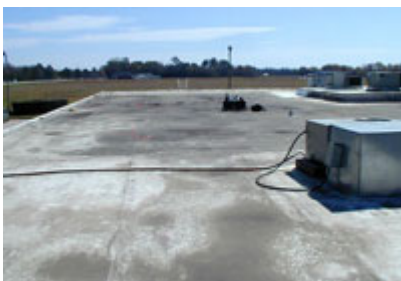
Photo 2: This photo shows the reality of a white roof surface membrane used in areas of heavy agricultural activity. The soil atop the membrane certainly has
