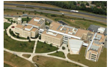
Photo 3: This ballasted roof system will provide greater benefits during its life than would a "cool" roof system that becomes soiled.
