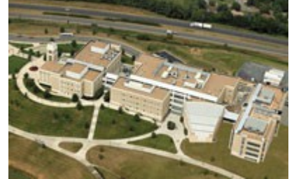
Photo 3: This ballasted roof system will provide greater benefits during its life than would a "cool" roof system that becomes soiled.
