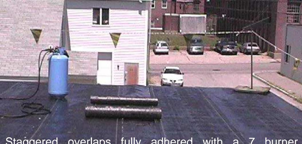
Staggered overlaps fully adhered with a 7 burner Stainless Steel Dragon Wagon, heat welded to form a watertight seal. The following link will take you to a YouTube video for a quick demo on how it is done. https://www.youtube.com/watch?v=jVOVW7zTYGo
