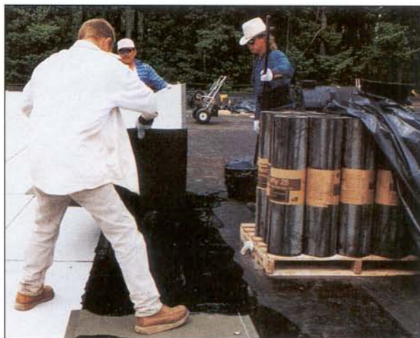
Photo 1: Two workers fly in a cap sheet onto a mopped substrate.
