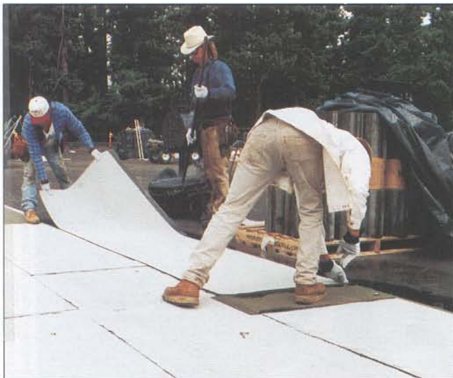
Photo 2: Workers, using the flying-in method, finish installing a cap sheet.
