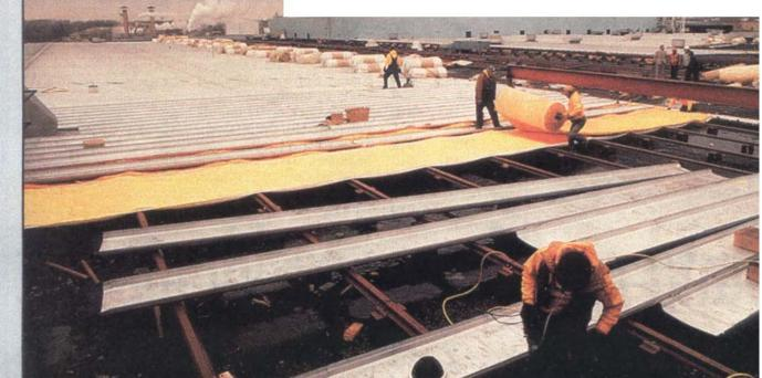
As the life-cycle cost study period is lengthened, there will be a shift to longer-lasting, lower-maintenance roofing systems.
