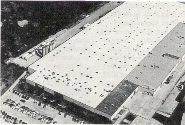
When rooftop penetrations are numerous, prefabricated flashings and membrane panels are most effective in protecting a structure against ponding water.
